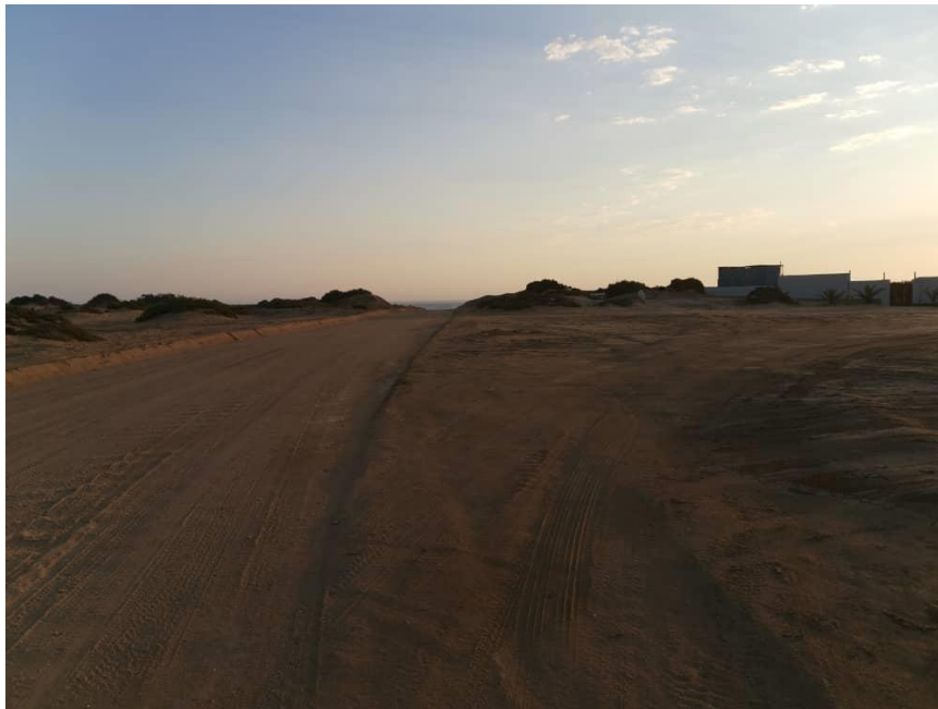
Figure 7: Existing access salt gravel road
