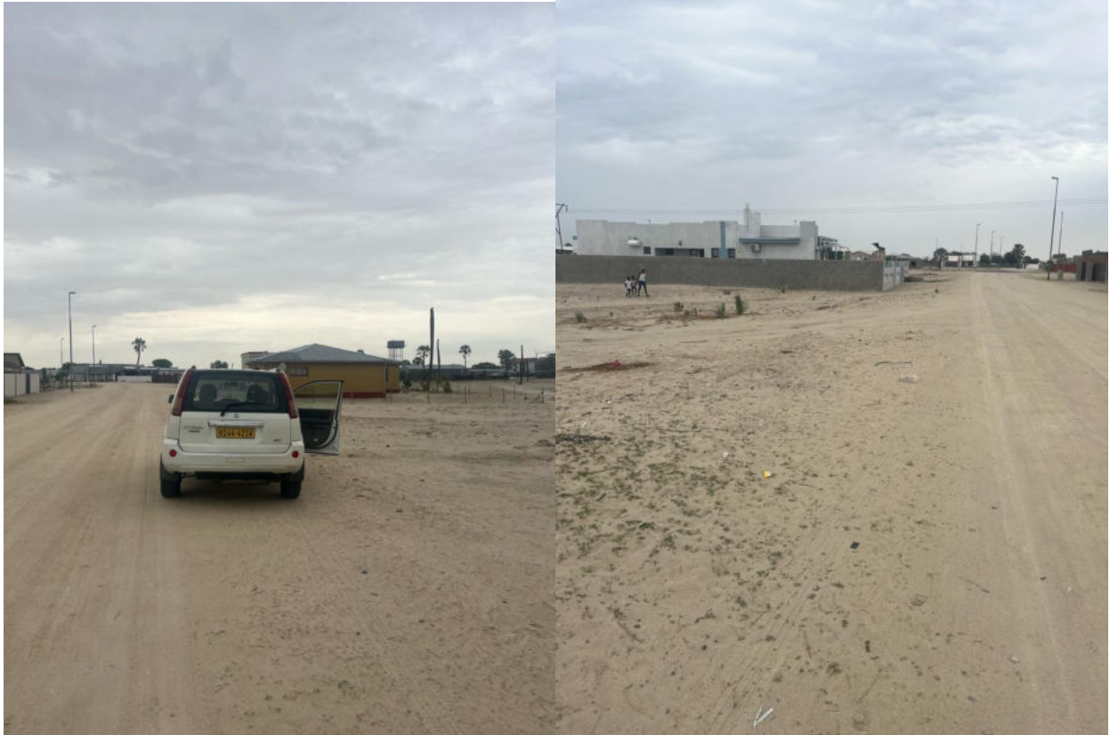
Figure 2: Typical conditions of Erven A-D/3571
