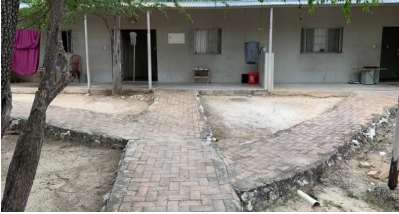
Figure 26. Paved pathways in the staff village.
