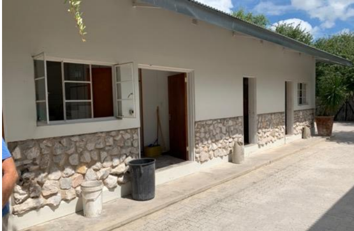
Figure 11. Storage shed with doors to laundry, store room and workshop.
