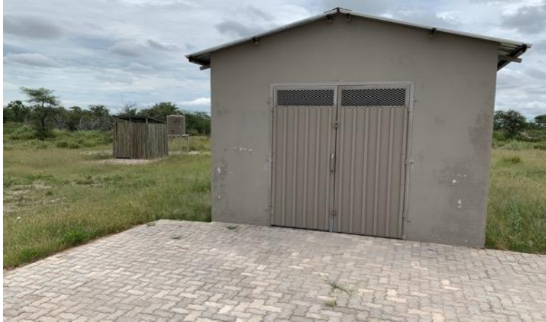
Figure 14. Shed for Avgas storage at the airstrip.
