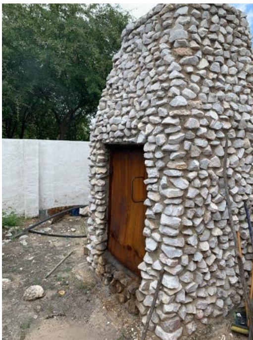
Figure 20. The incinerator enclosure is inaccessible to mammals.
