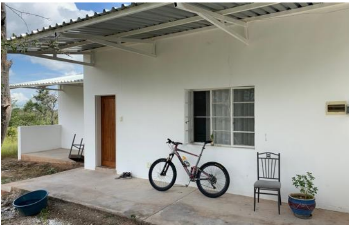
Figure 12. The manager's house has two en suite bedrooms.
