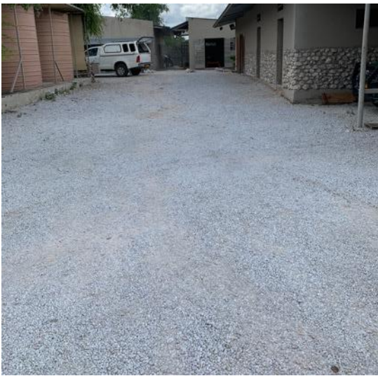
Figure 30. Gravel surface in the back-of-house.
