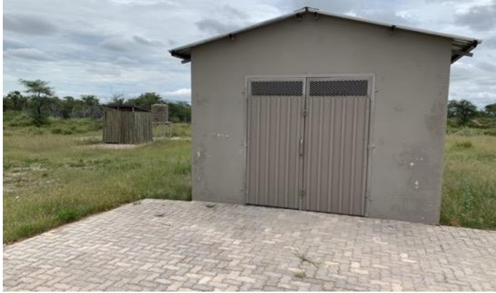
Figure 18. Store room for Avgas at the airstrip. The toilet is visible in the background.
