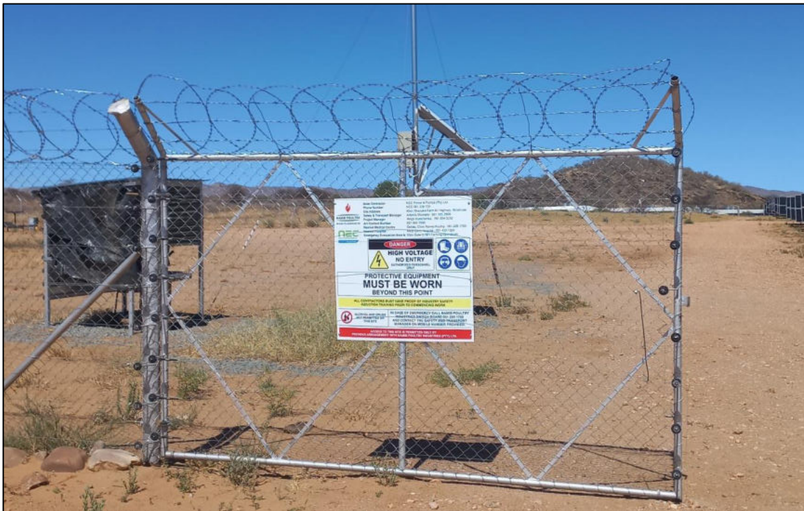
Figure 7: Entrance to Solar Plant
