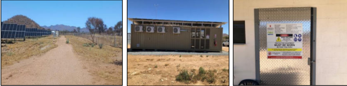
Figure 6: Photos after construction of solar site
