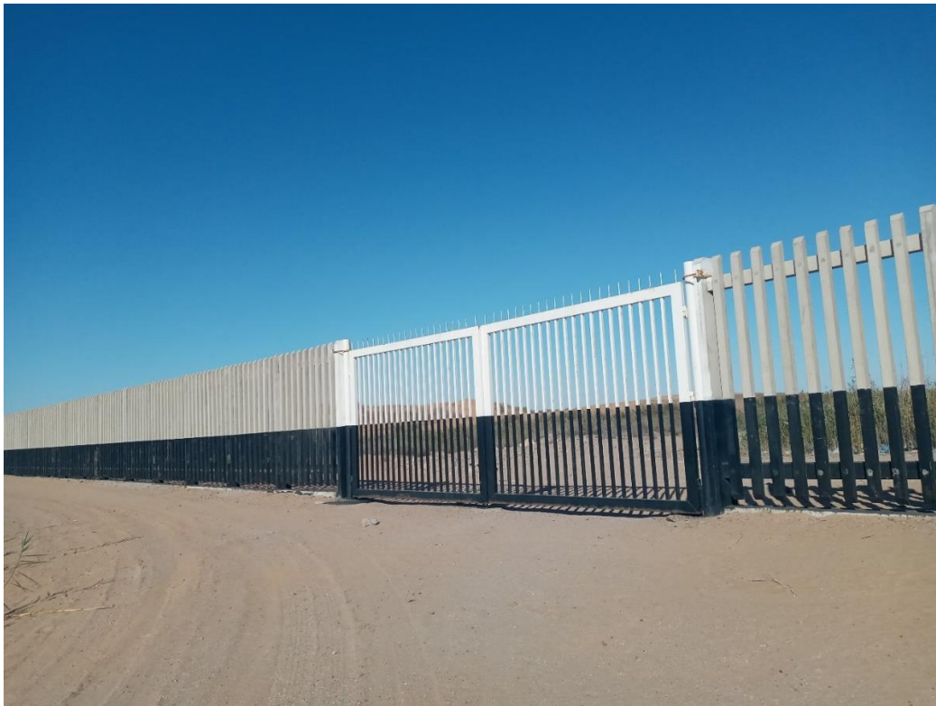
Figure 2: Completed fence at the entrance of the landfill site, phase 1 and 2
