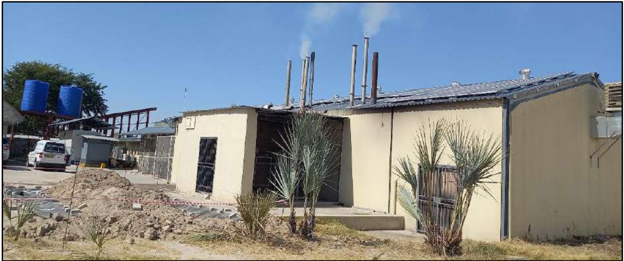
Figure 6: Project Footprint - Looking SE
