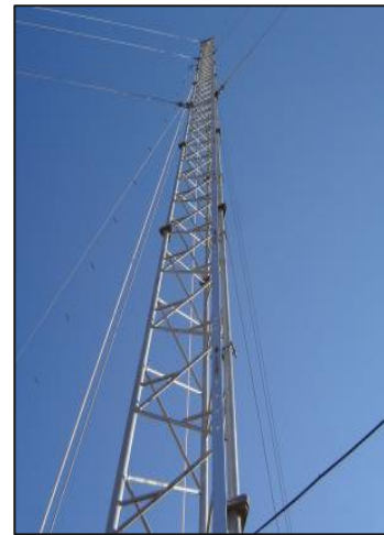
Photo 2-1: Example of a guyed structure.
