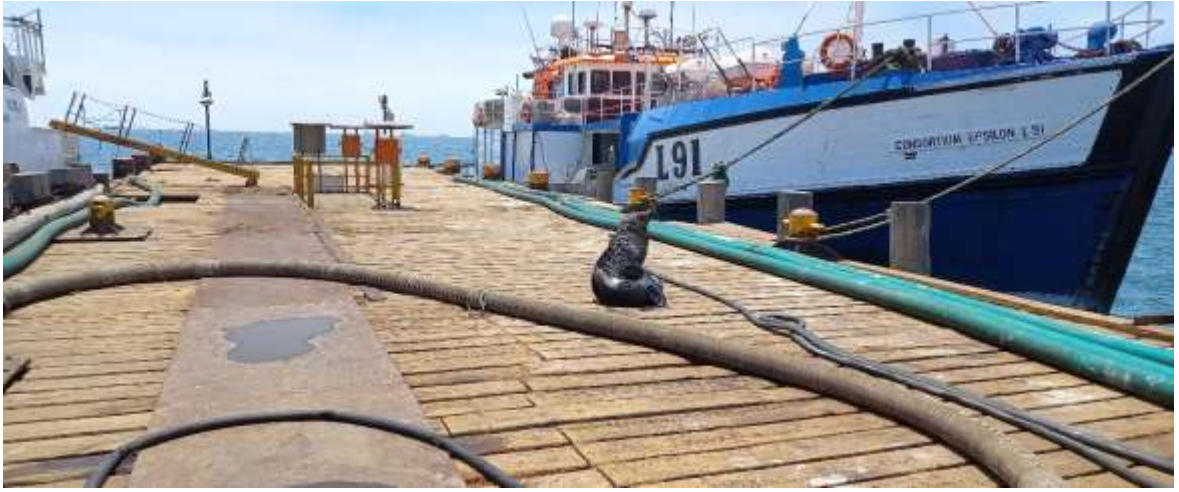
Figure 13: A Seal taking a break on the Jetty to be demolished
