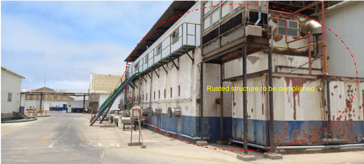
Figure 11: Redundant Building to be Demolished
