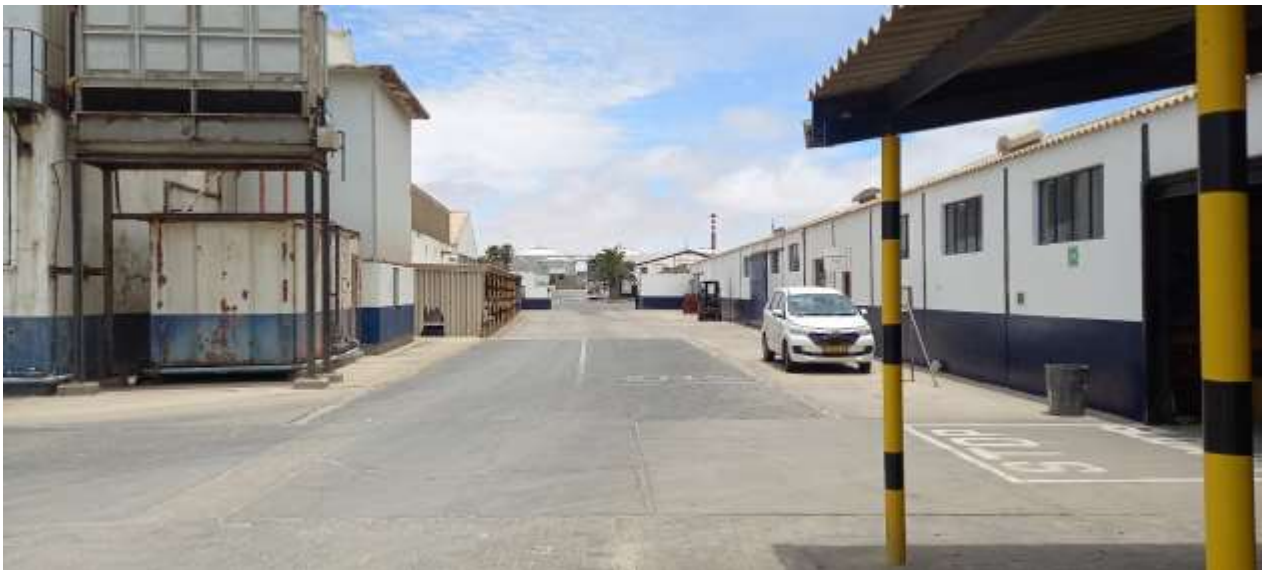
Figure 5: Entry and Exit Point to the Proposed Site with fuel storage tanks in the background
