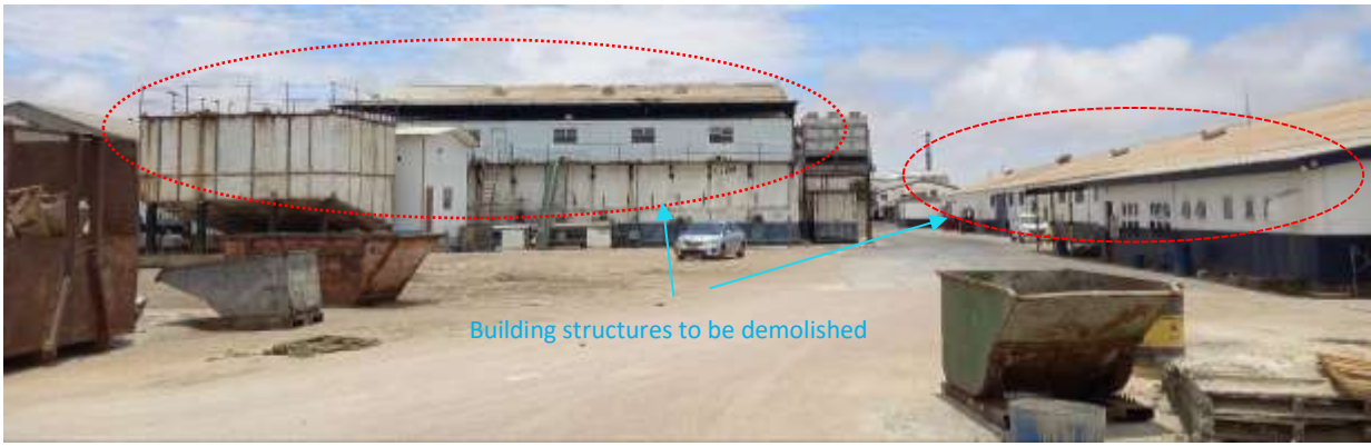
Figure 10: Building Structures to be Demolished
