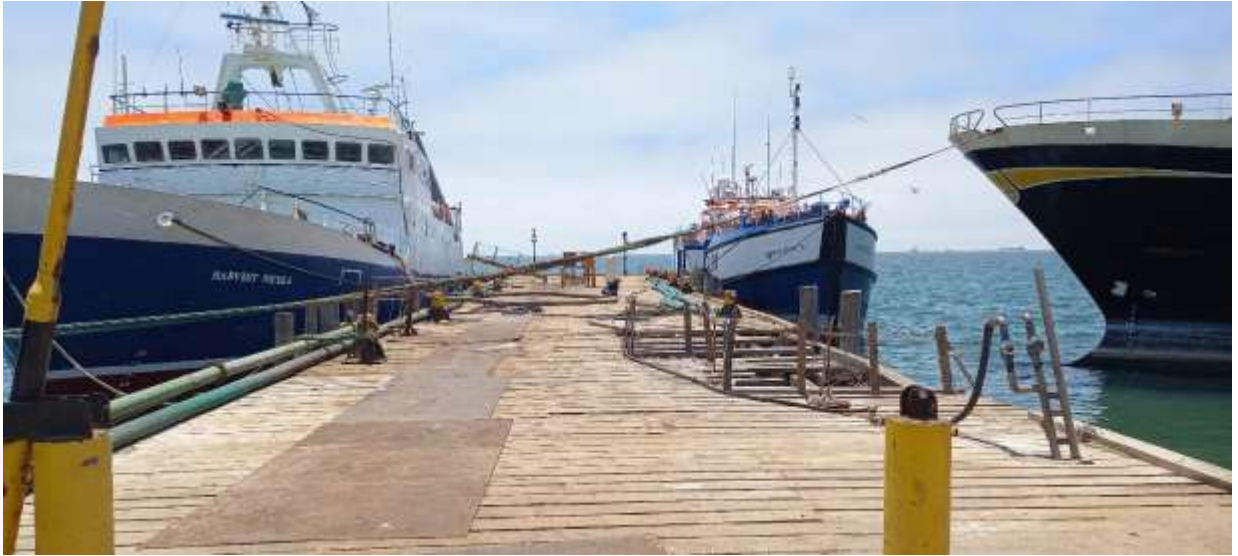
Figure 7: Existing Wooden Jetty to be Demolished
