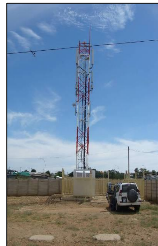
Photo 2-1: Example of a lattice structure.
