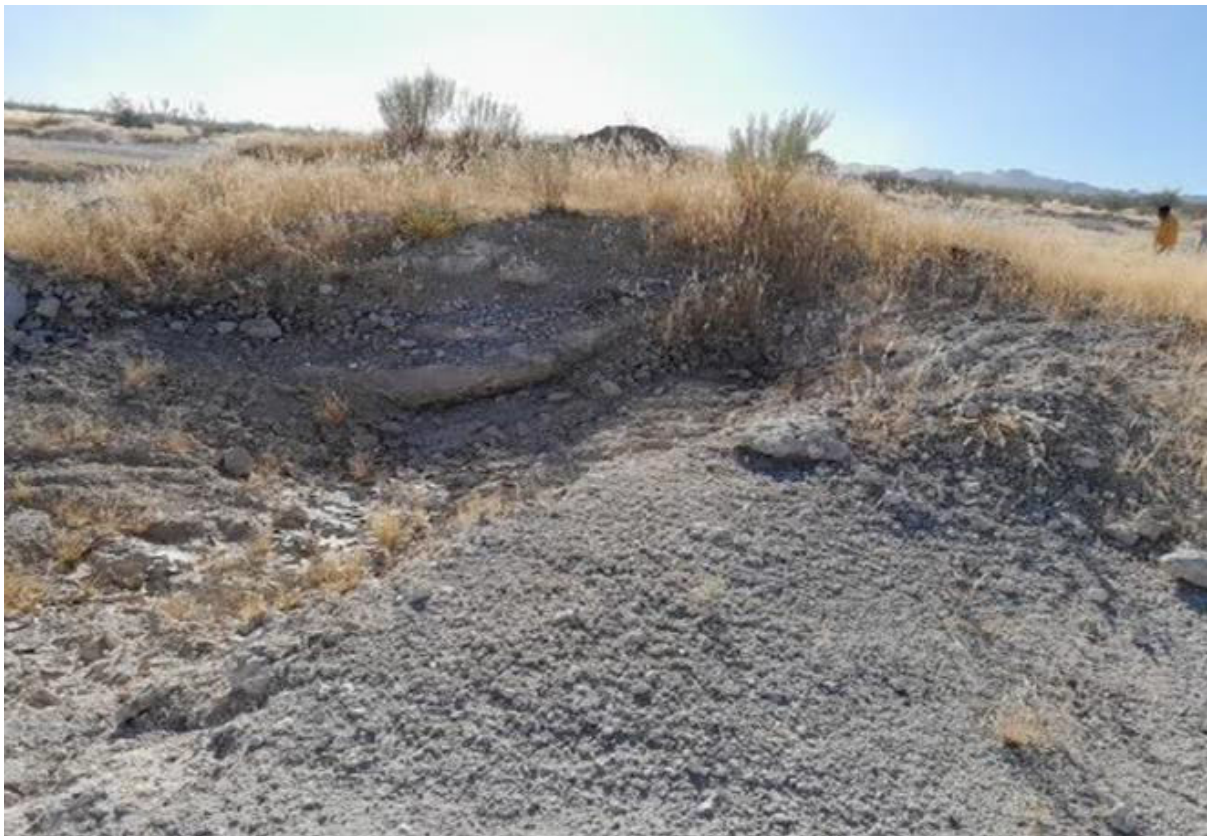
Picture 1: Unrestrained excavation resulting in gullies
