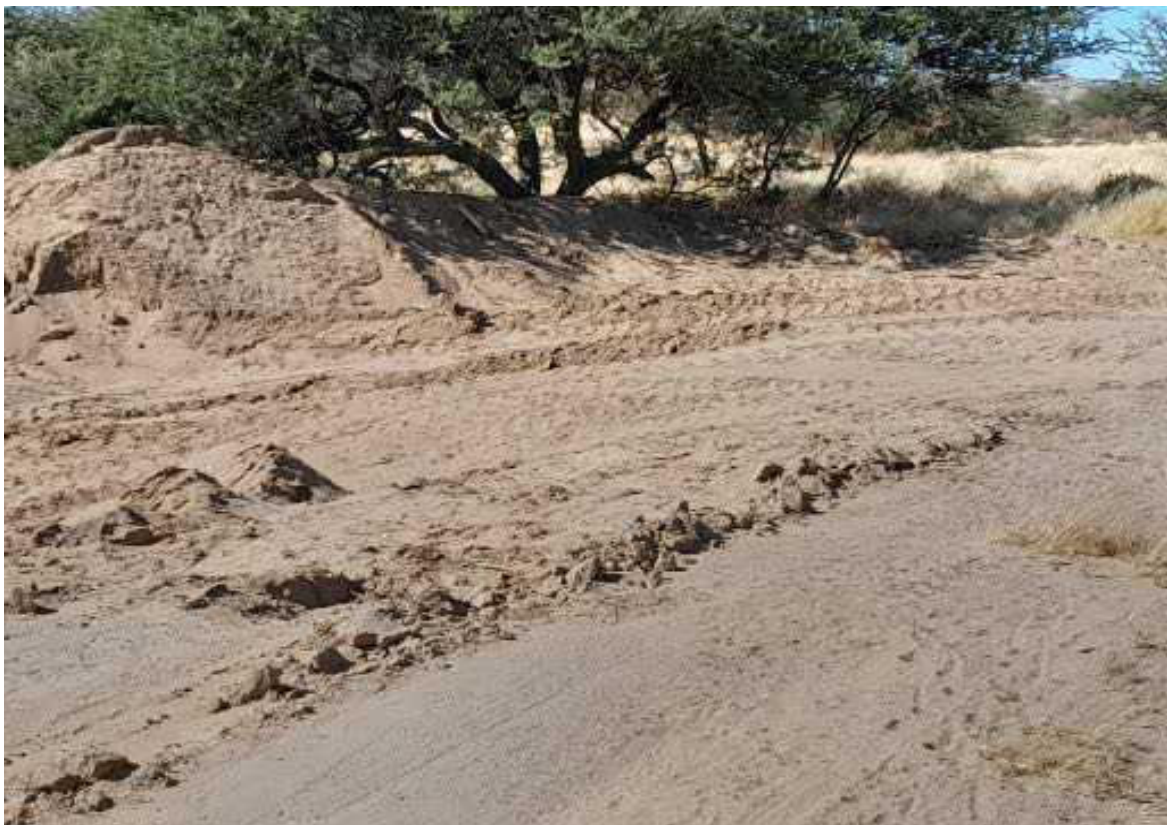
Pic 5: Uncontrolled excavation across road path
