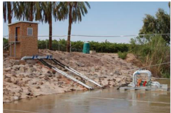
Option 2: A floating pontoon
