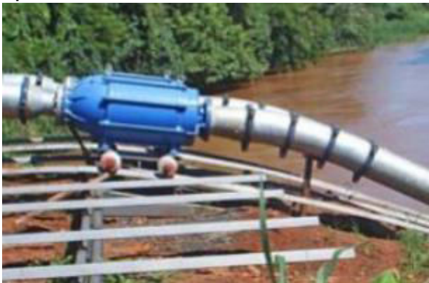
Option 3: Pumps on rails
