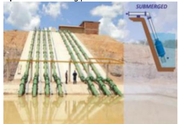
Option 4: Submerged in-line pumps fixed to the embankment abstraction works
