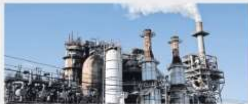
The LyondellBasell refinery, located near the Houston Ship Channel, is seen in Houston, Texas, U.S., May 5, 2019. PHOTO REUTERS/LOREN ELLIOTT
