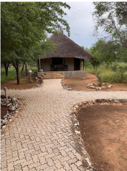
Figure 12. Paved pathways to carry foot traffic.
