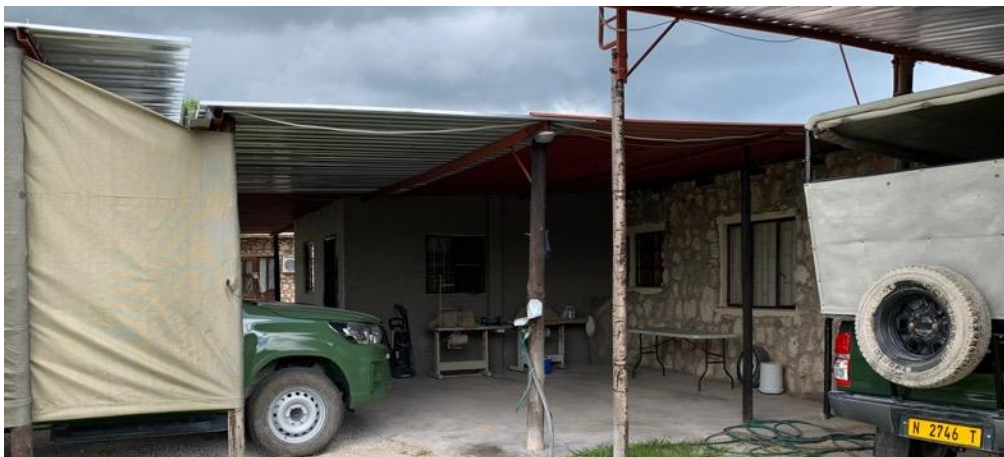
Figure 33. Vehicle shed and a stone house in the game drive complex.
