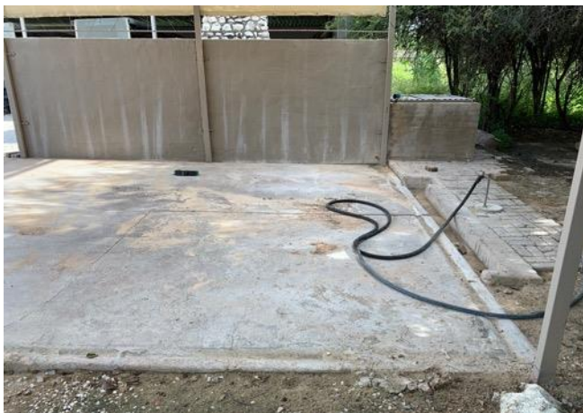
Figure 27. The car wash area with sloping floor and drainage ditch.
