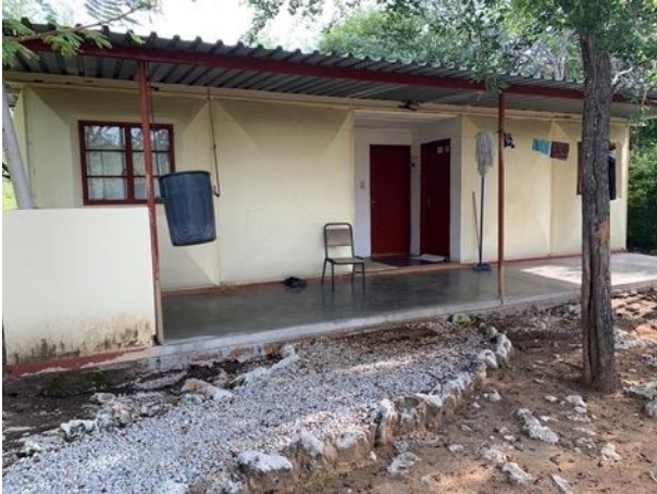
Figure 13. A staff village block with two bedrooms, a bathroom and veranda.
