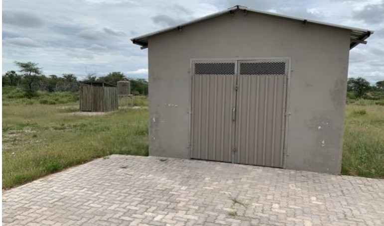
Figure 29. Afgas shed. Toilet and water tank are visible on the left.
