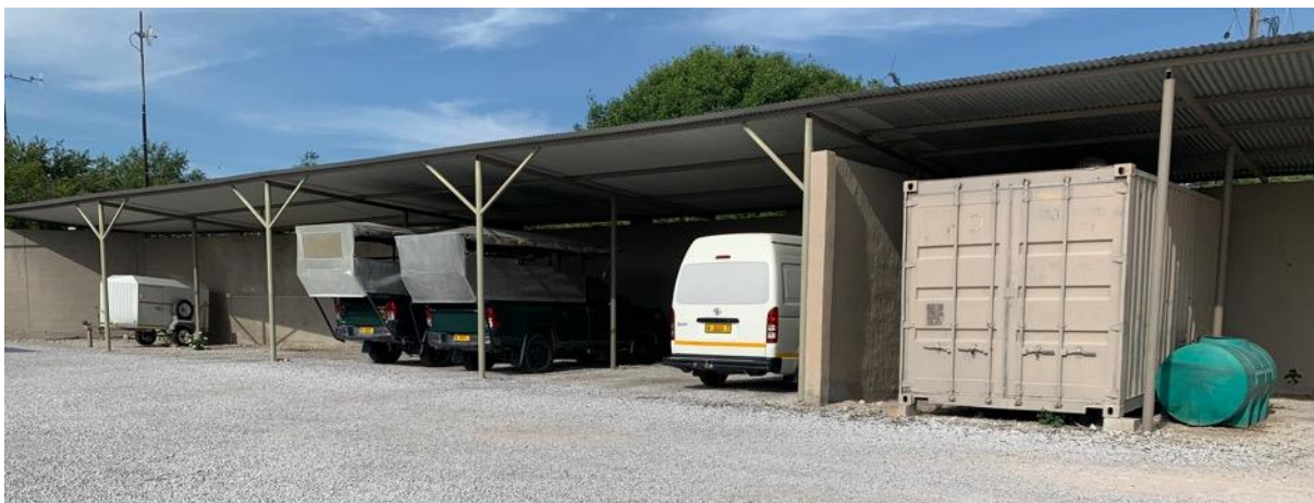
Figure 25. Carport with 12 parking bays.
