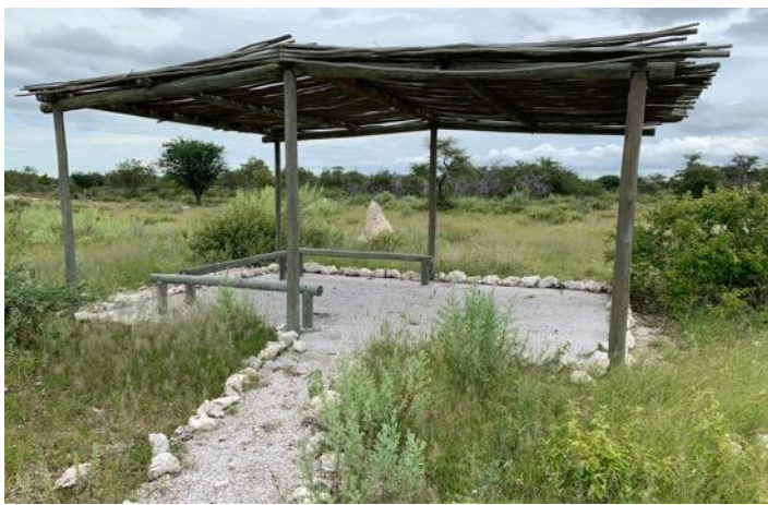
Figure 30. Shaded waiting area with gravel floor.
