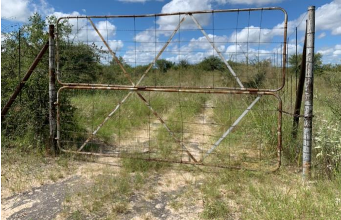
Figure 43. Gate to the fenced in farm landfill.
