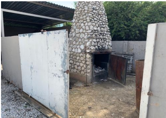
Figure 42. The incinerator, secured by high walls and a sliding gate.
