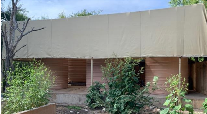
Figure 34. Six water tanks.
