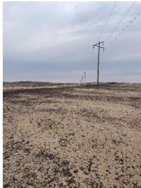
Figure 3: Existing 22KV OHL and cleared servitude
