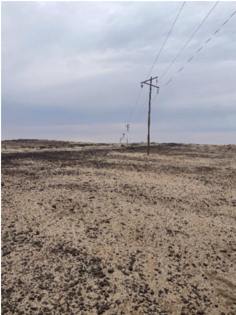
Figure 3: Existing 22KV OHL and cleared servitude
