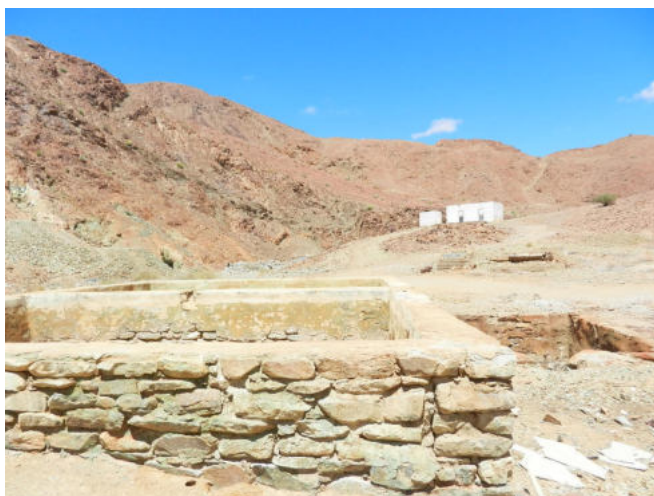
Photo 4: Remains of the old mine infrastructure and leach tanks within the Volstruis River
