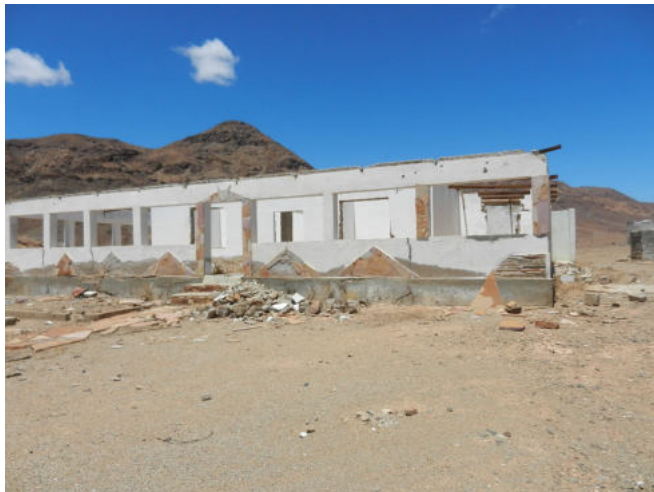
Photo 3: The remains of the old, dilapidated Tsams Farm house on the banks of the Haib River.
