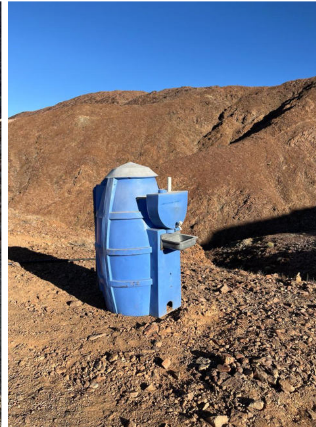
Plate 10 : Ablution facilities installed
