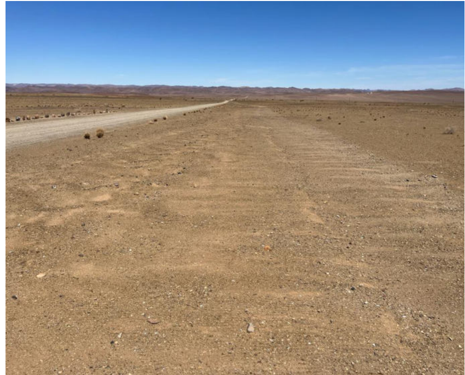
Plate 6 : Rehabilitation of old tracks
