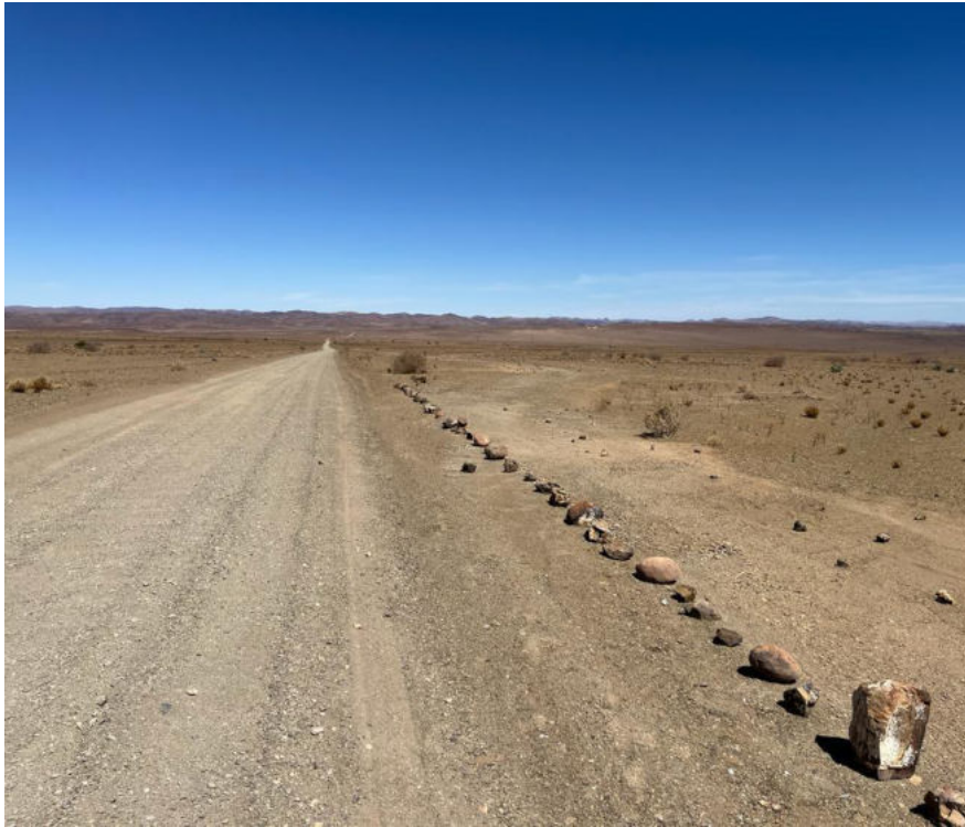
Plate 5 : Measures to prevent off roading and improve track discipline
