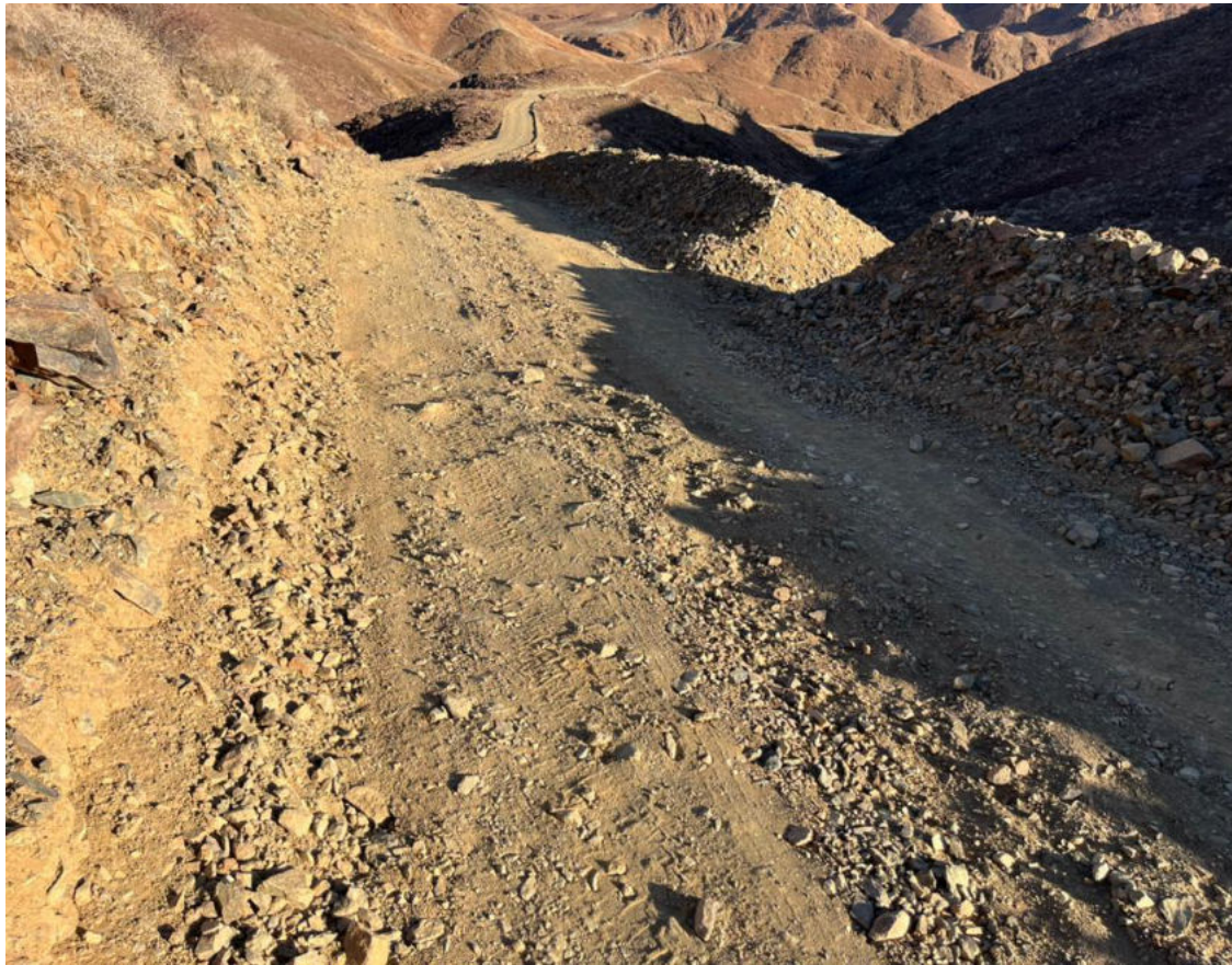
Plate 9 : Physical measures to prevent erosion on steep roads
