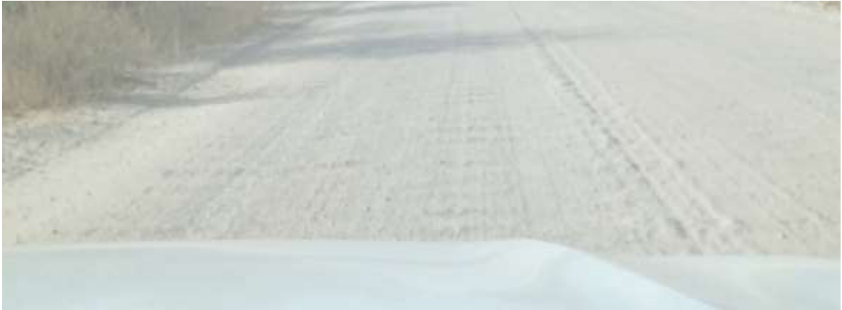
Figure 4: A Corrugated Section of C38
