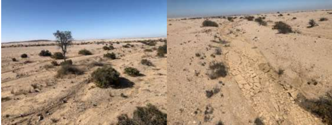
Figure 6-6: Evidence of active flow on the surface drains
