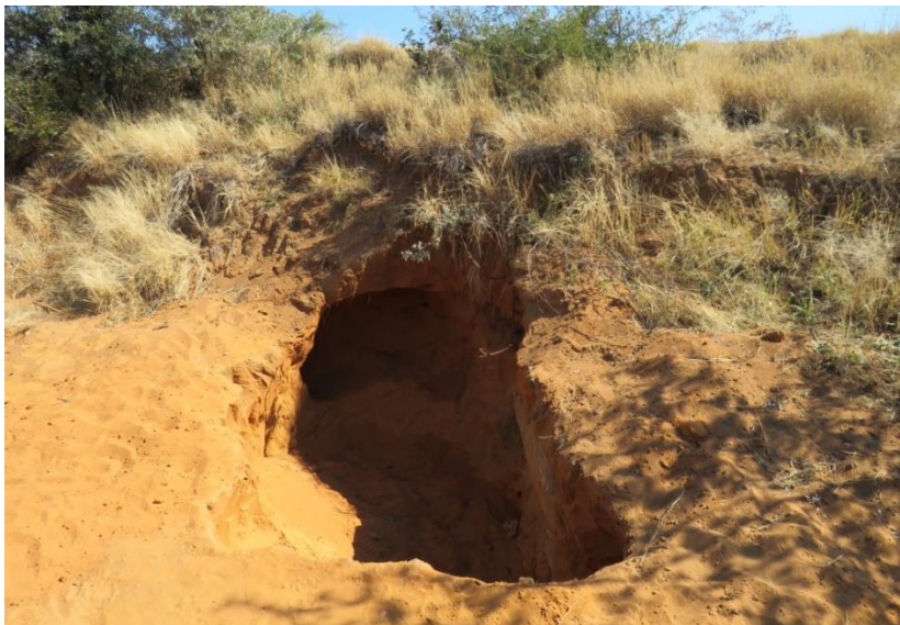
Figure 4. Illegal soil excavation adjacent to the railway embankment
