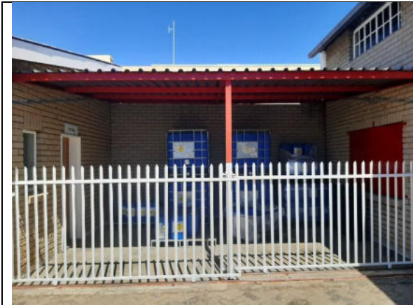
Photo 4-1 Hydrogen peroxide storage
