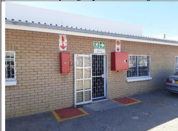
Photo 4-3 Firefighting equipment and signage
