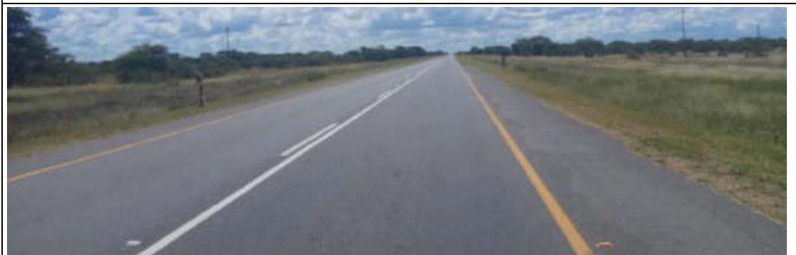
Figure 15: Top & Below – View along B1 and from the Site to Omatako Mountains
