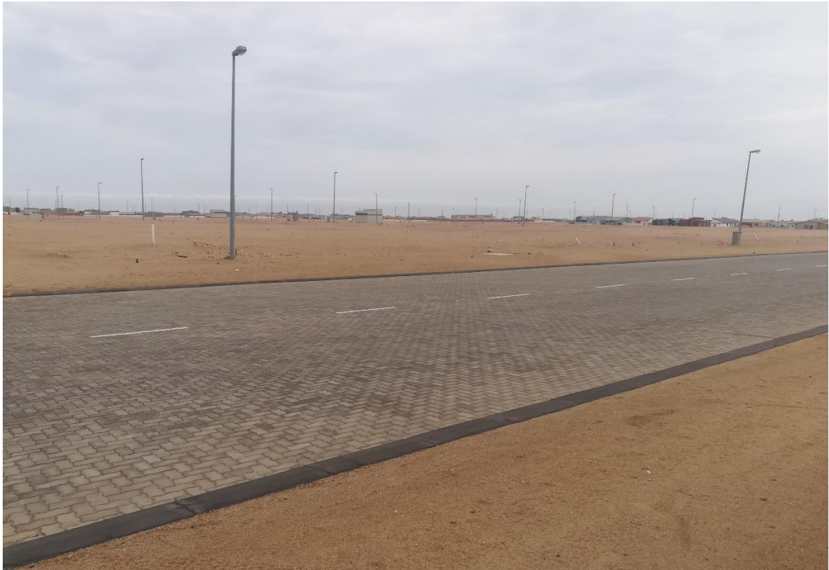
Figure 7 Serviced Extension of Matutura
