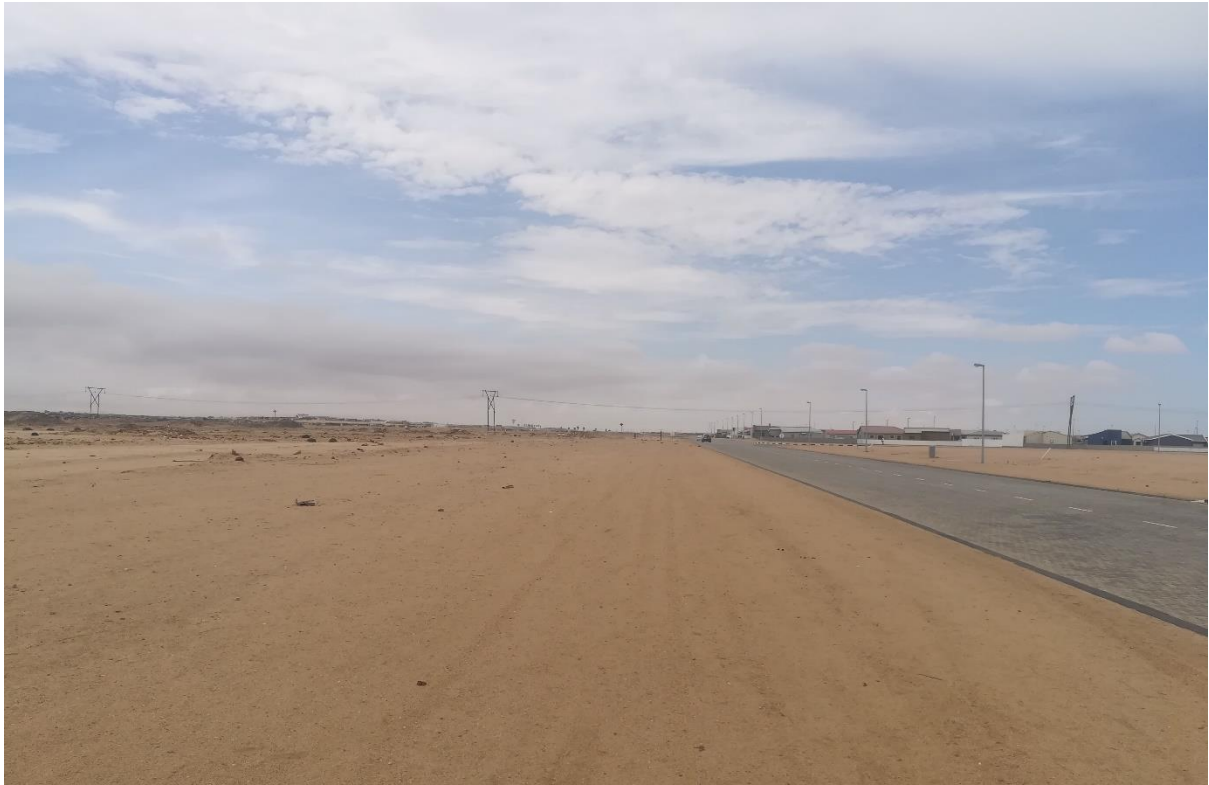
Figure 5 Un-serviced portion on the left and serviced portions of Matutura Extensions on the right
