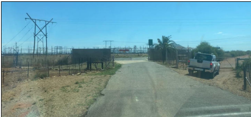
Image 1-6: Entrance to Nampower substation (straight ahead) and new entrance to PV Plant (to the right)
