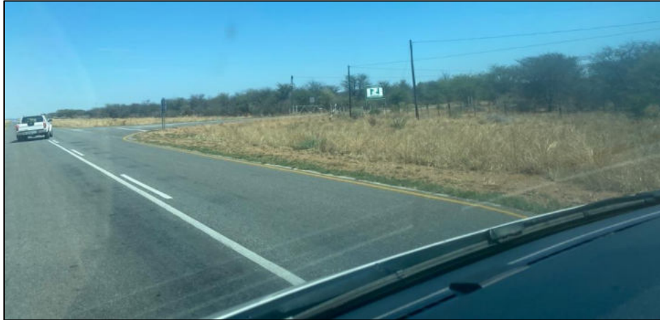
Image 1-4: B1 approach to Gerus Substation turnoff
