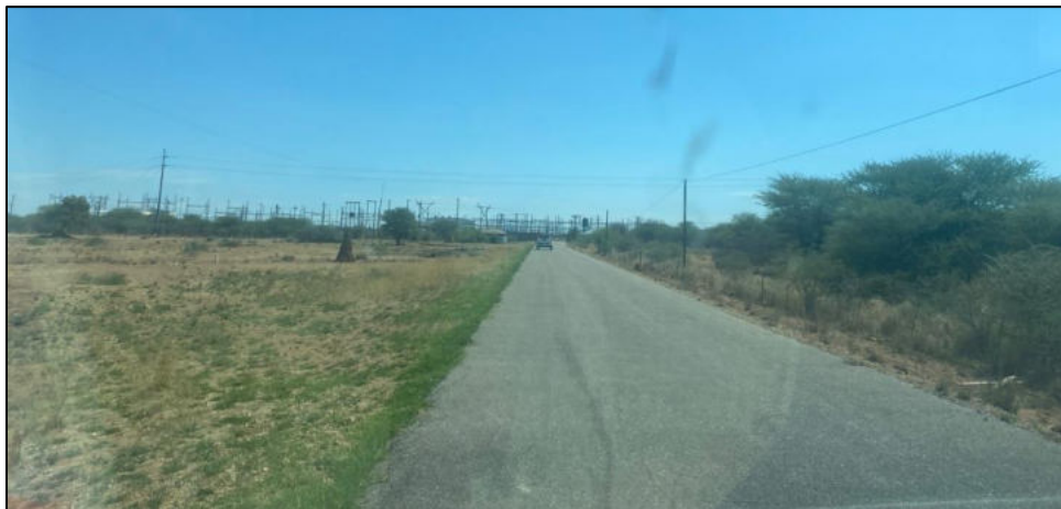
Image 1-5: Paved access from B1 turnoff
