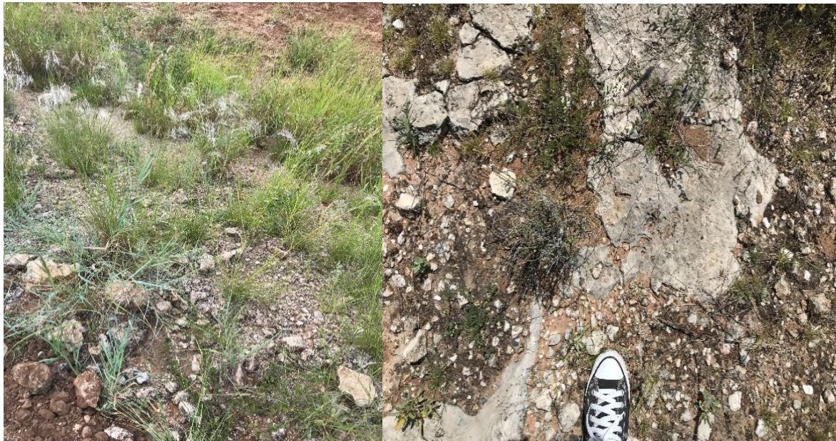
Figure 13: Exposed weathered and fractured quartzite’s at proposed site
