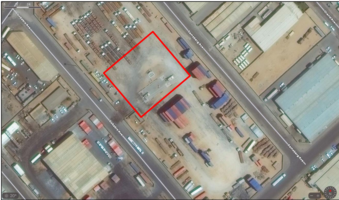
Figure 7: Photo showing locality of diesel tanks
