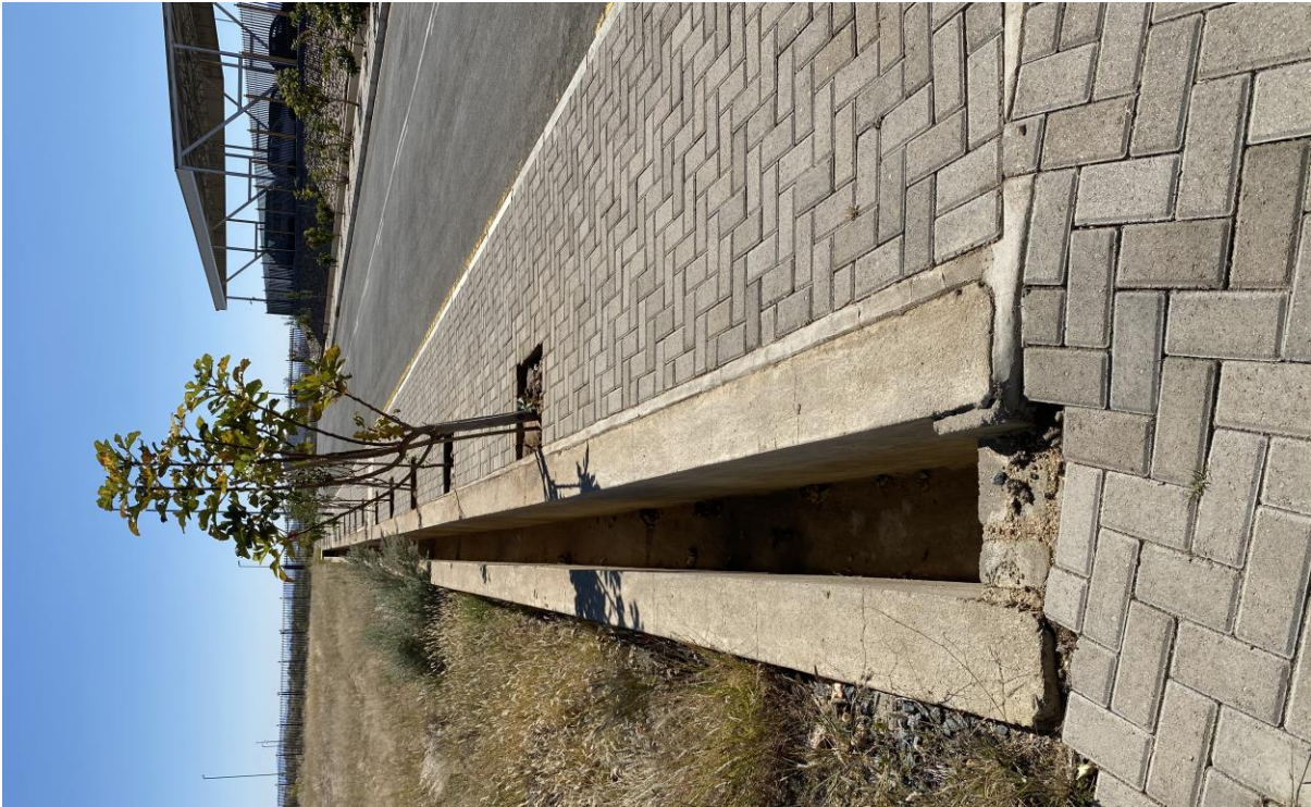
Figure 2.5: Stormwater drainage system
