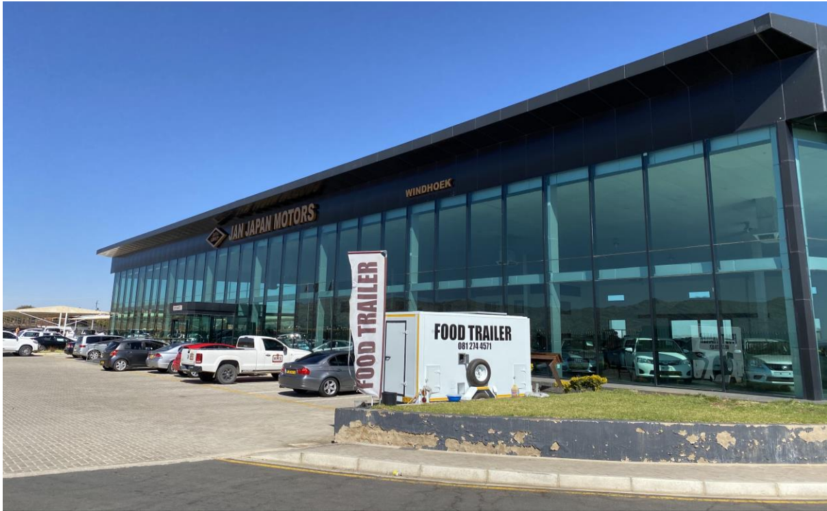
Figure 2.2 Current view of the Jan Japan Motor Dealership - Brakwater
