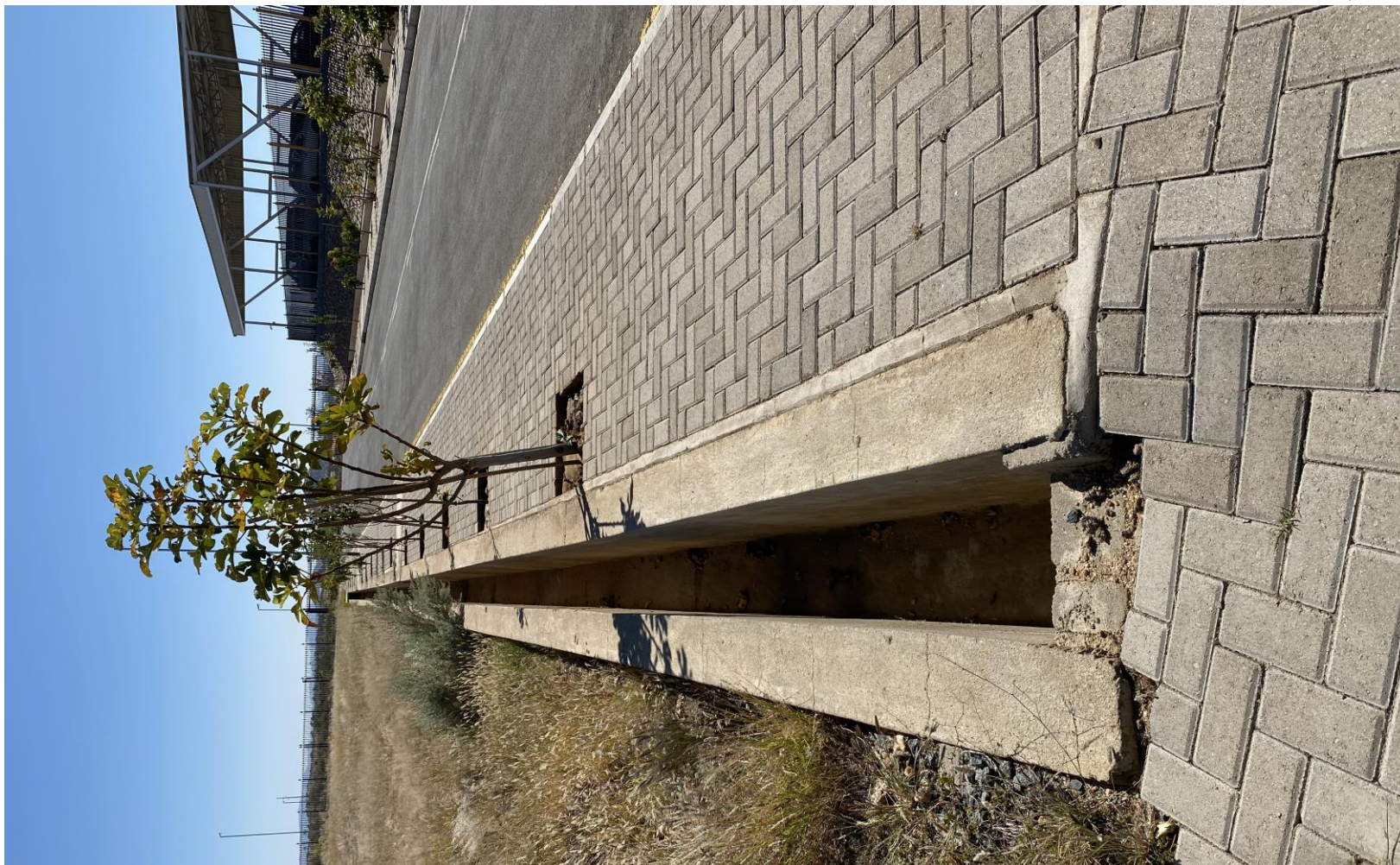
Figure 2-5: Stormwater drainage system
