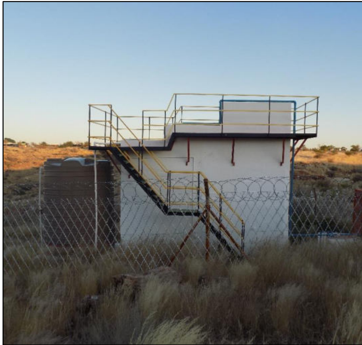
Figure 1-3: Wastewater Treatment Plant
