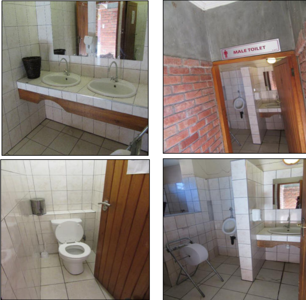
Figure 1-3: Ablution facilities on site
