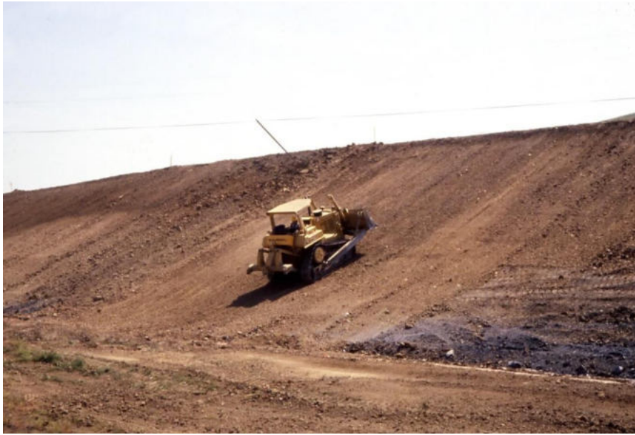
Figure 2. Illustration of the 1:3 slope fall
