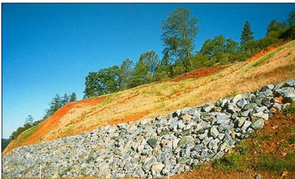
Figure 3. Rock buttress illustration
