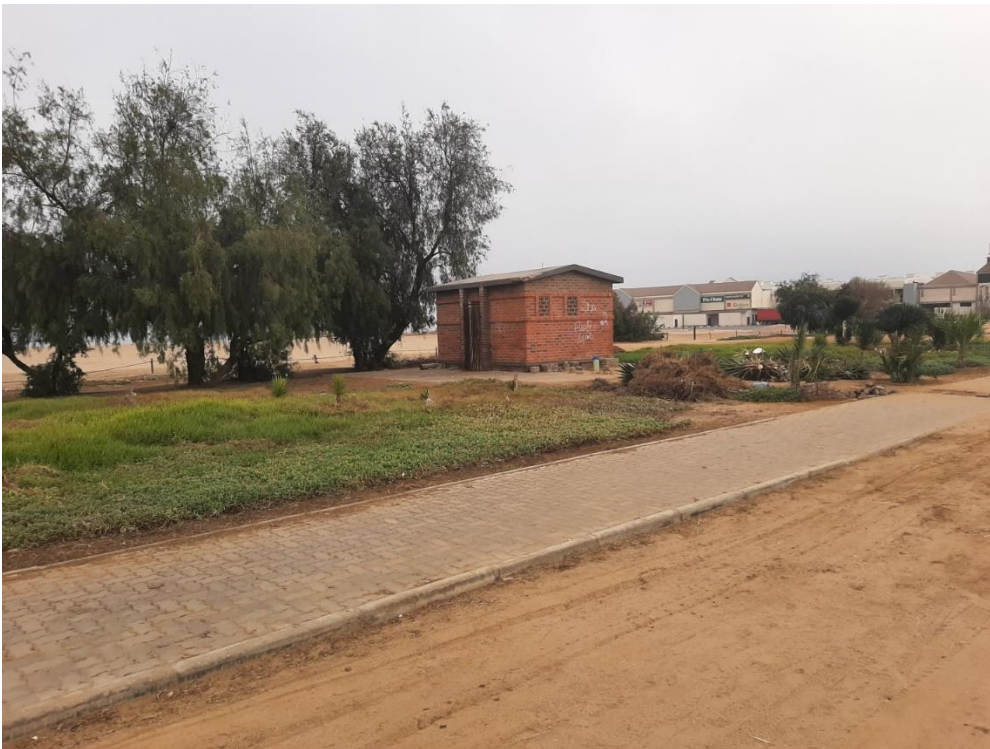
Figure 6: Example of the existing toilet facility
