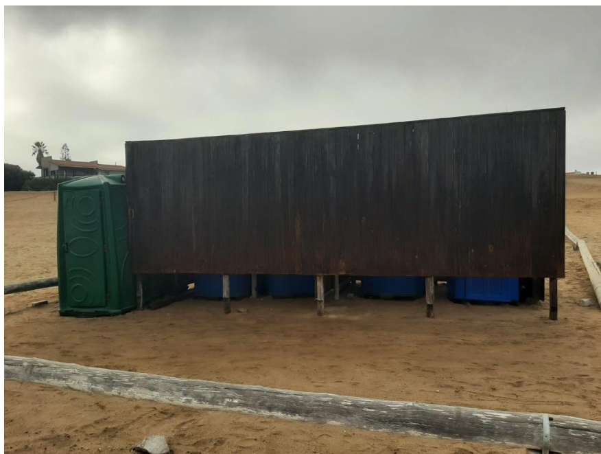
Figure 10: Existing “OK Parking” temporary toilet facility
