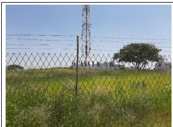
Photo 1. Project area and view to the north
