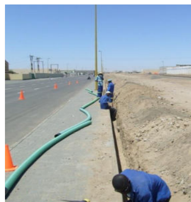
Figure 4: Fibre optic cables are put in trenches in the existing road reserve.
