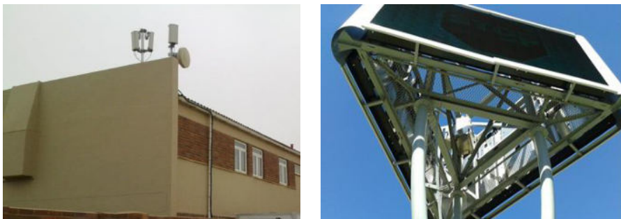
Figure 1: Example of equipment on existing structures (left - on top of a building) (right - inside a billboard). Photos from MTC.
