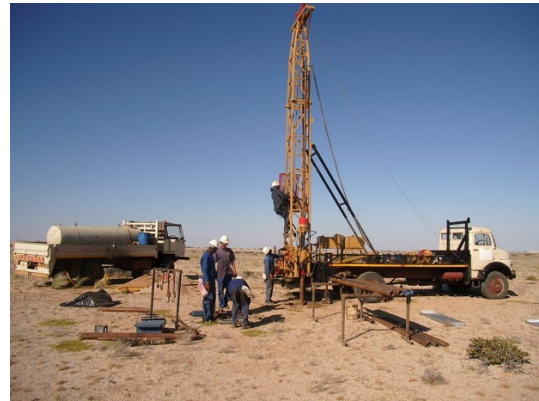
Figure 3-3: Example drill rig
