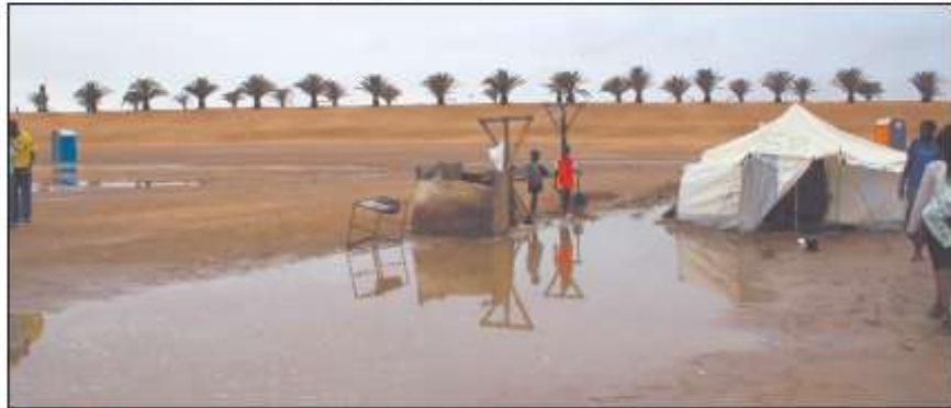
Underwater... Several homes, including the temporary campsite of Otweya, housing last year's fire victims, were flooded during a flash flood on Saturday evening at Walvis Bay. There was also considerable damage to electric appliance and other valuable items of residents. Photo: Estuine de Klerk
