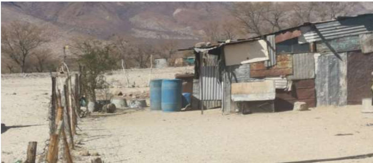
Figure 7: Temporary accommodation facilities for SSMS
