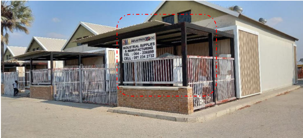
Figure 23: View of the Front Porch of Unit 4
