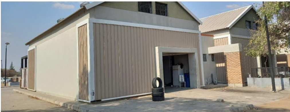
Figure 21: View of Unit 4 from the South
