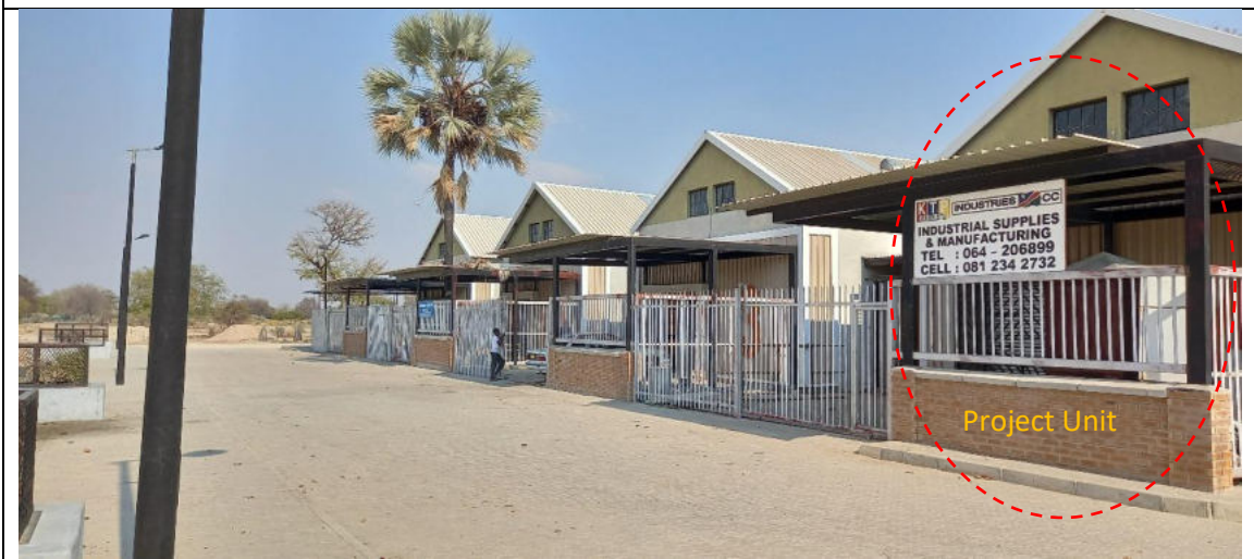
Figure 5: View of All Four Industrial Units Seen from NW
