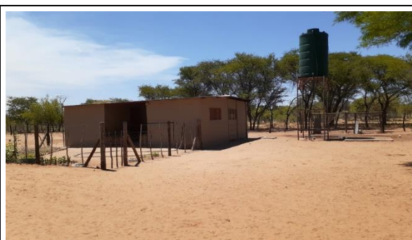
Photo 4-17. Water storage at labour accommodation area
