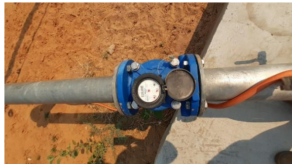
Photo 4-11. Flowmeter installation at Ohlshagen No. 174 (Portion 2)
