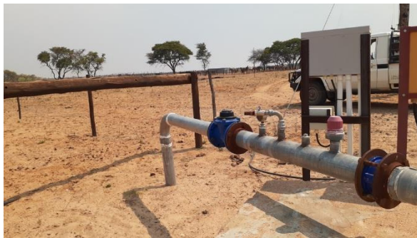
Photo 4-10 Typical borehole installation on Ohlshagen No. 174 (Portion 2)
