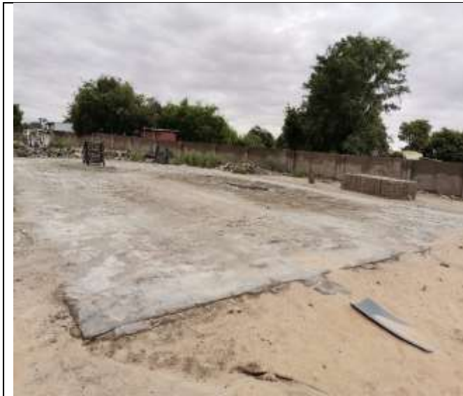
Boundary wall onsite
