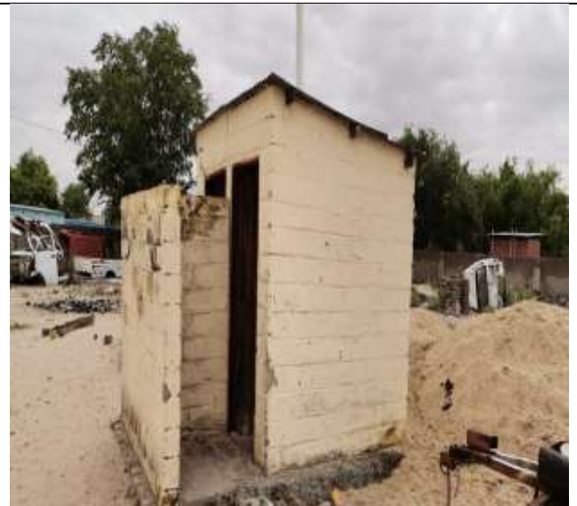
Ablution facilities for employees & customers
