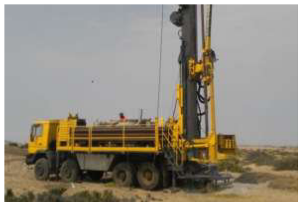
Figure 10: A Truck Mounted RC Drill Rig
