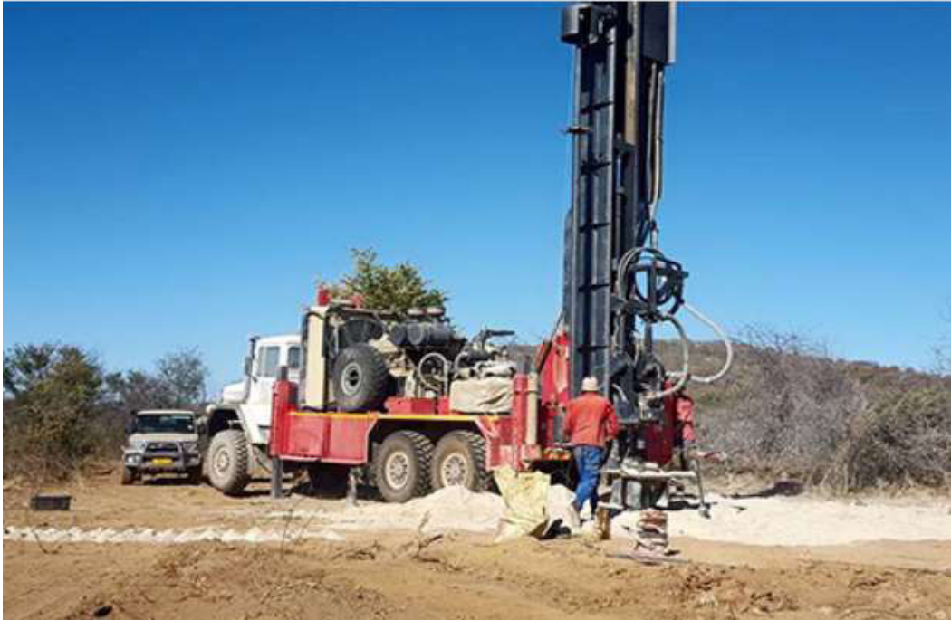
Figure 8: Vegetation Clearing Around a Drilling Site (Source: African Drilling)
