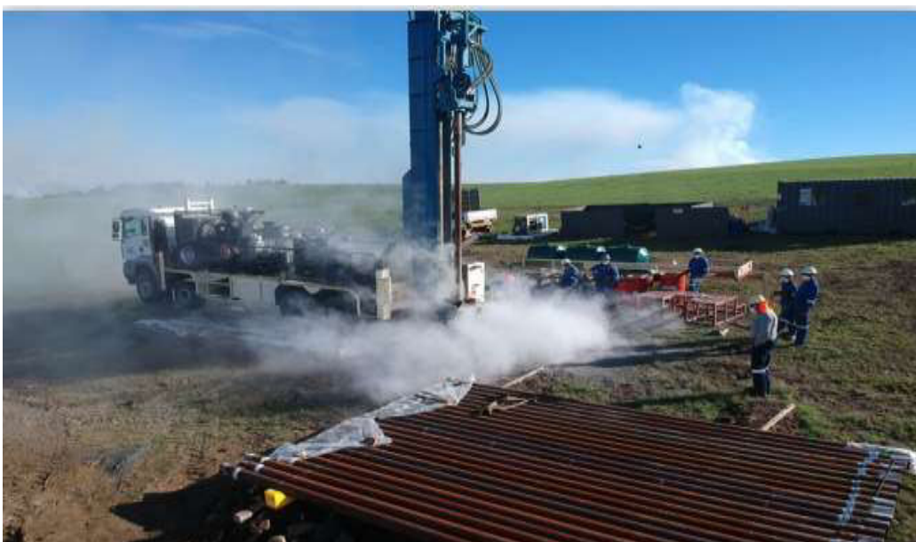
Figure 7: Dust Generated During Drilling Activities (Source: torqueafrica.co.za)
