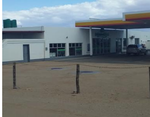
Photo 2. Existing underground storage tanks
