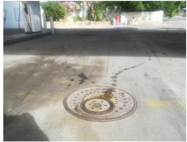
Photo 4. Existing forecourt and USTs
