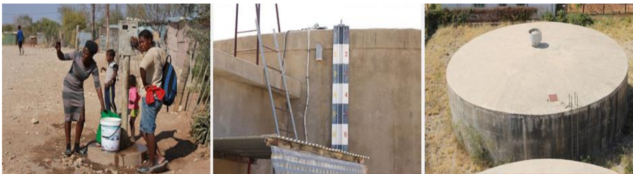
Pictures 1-3: Community Prepaid Water Standpipe in Informal Settlement Area. 50 Standpipes installed in this area. Water Tower with 2 Reservoirs supplying water to the town.
