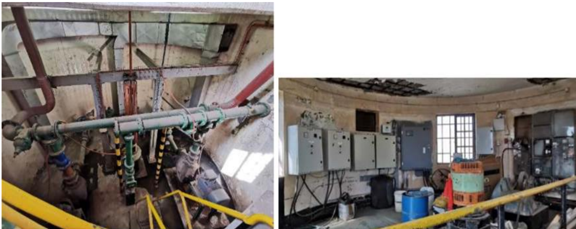
Figure 10.4: Mechanical/electrical condition of Kuisebmond existing pump station
