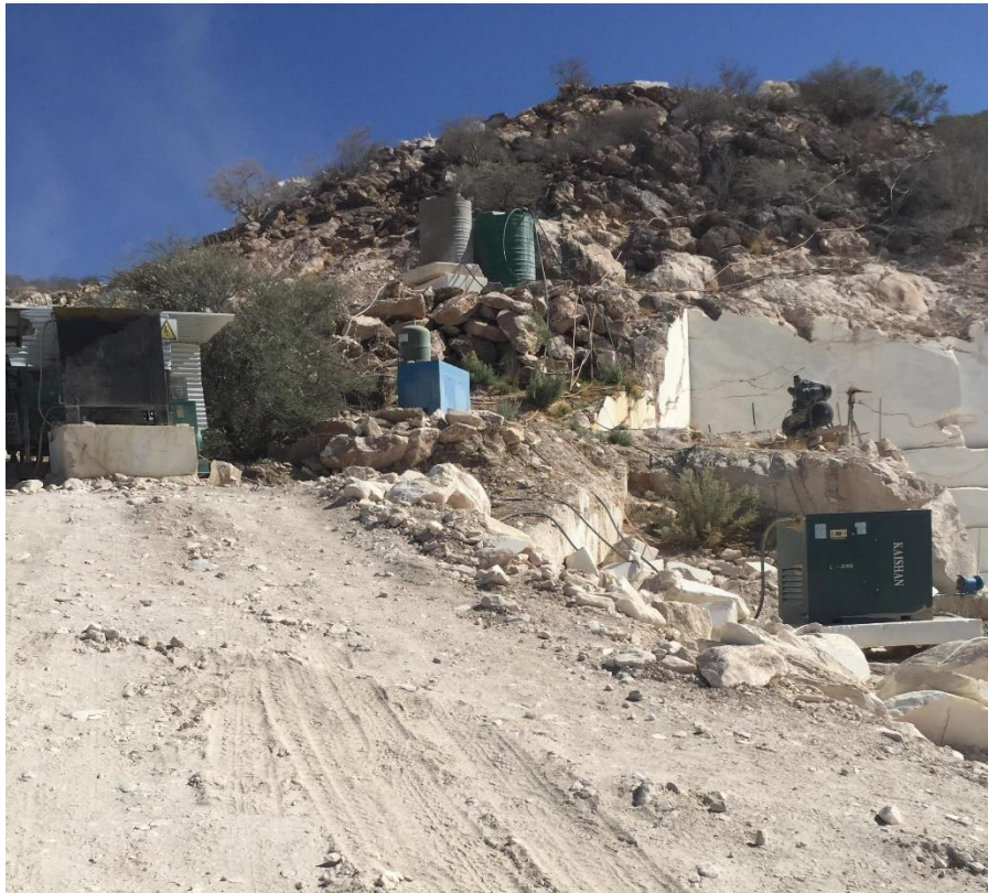
Figure 8: Water tanks and diesel-powered generator
