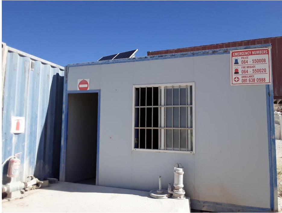
Figure 7: Store room, emergency contact details, and firefighting equipment
