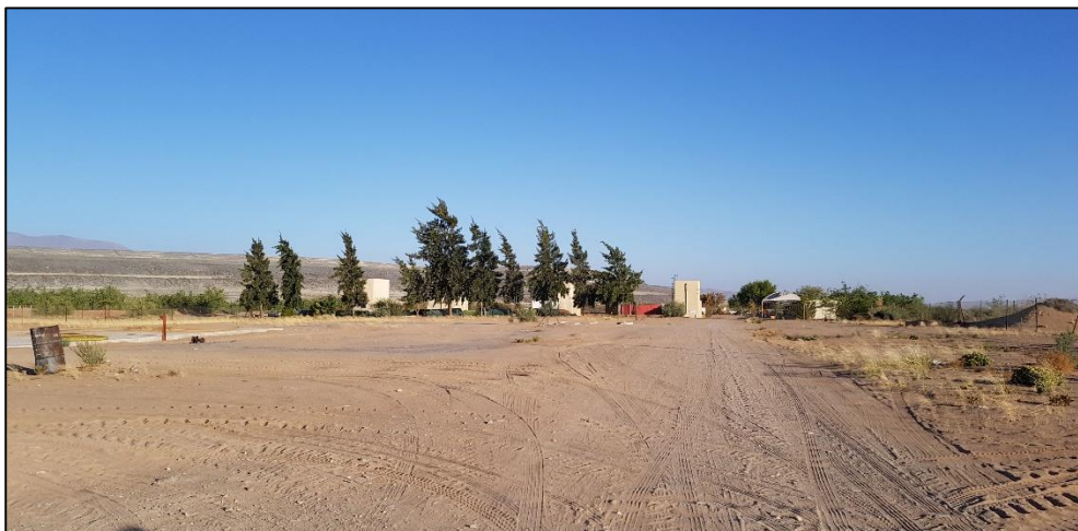
Figure 2: View of the Sewage Treatment Plant site
