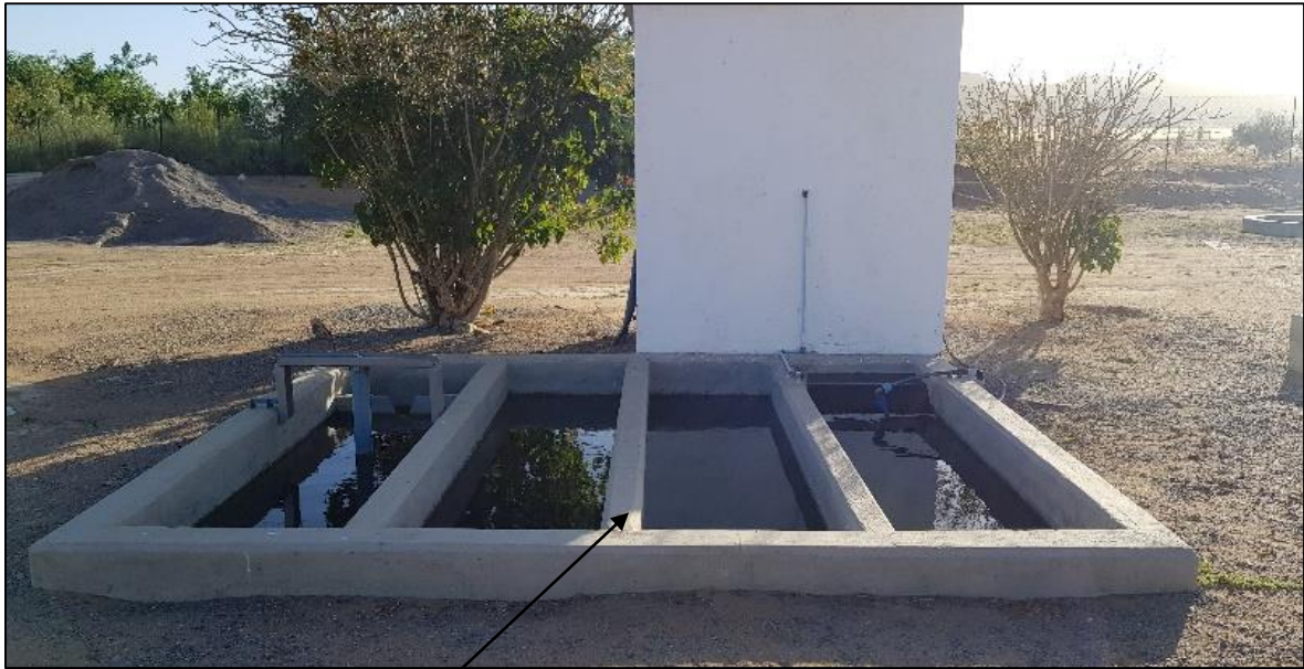
Figure 8: Chlorine dosing dams
