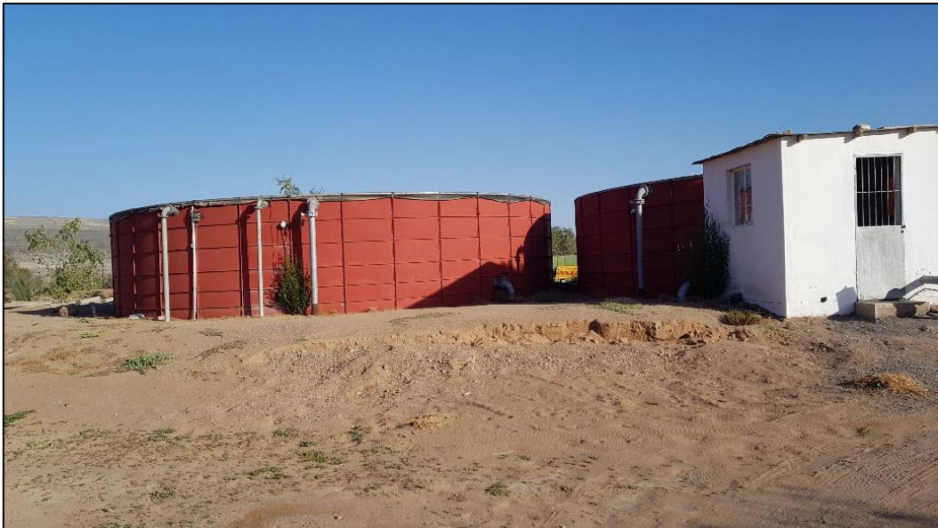
Figure 7: Storage Tank for treated water
