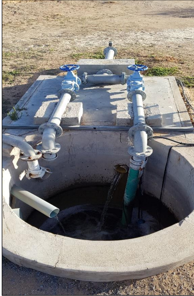
Figure 6: Treated water collection point
