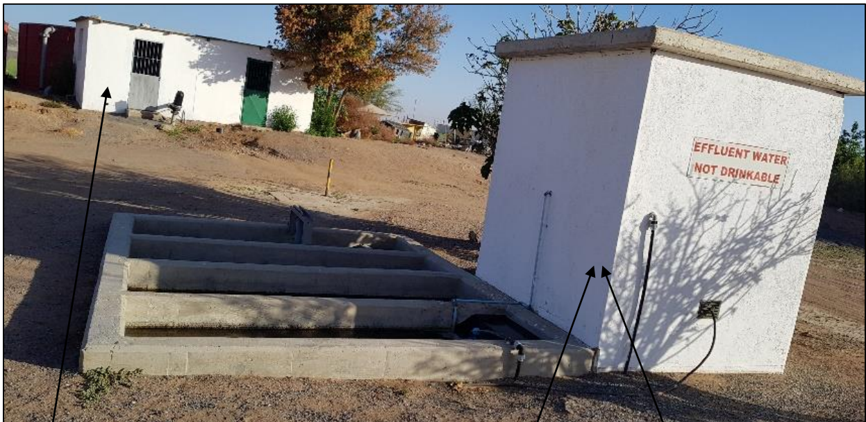
Figure 9: Chlorine contact room & Pump station room
