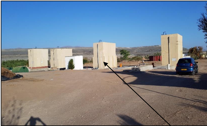
Figure 3: Trickling Filter Towers
