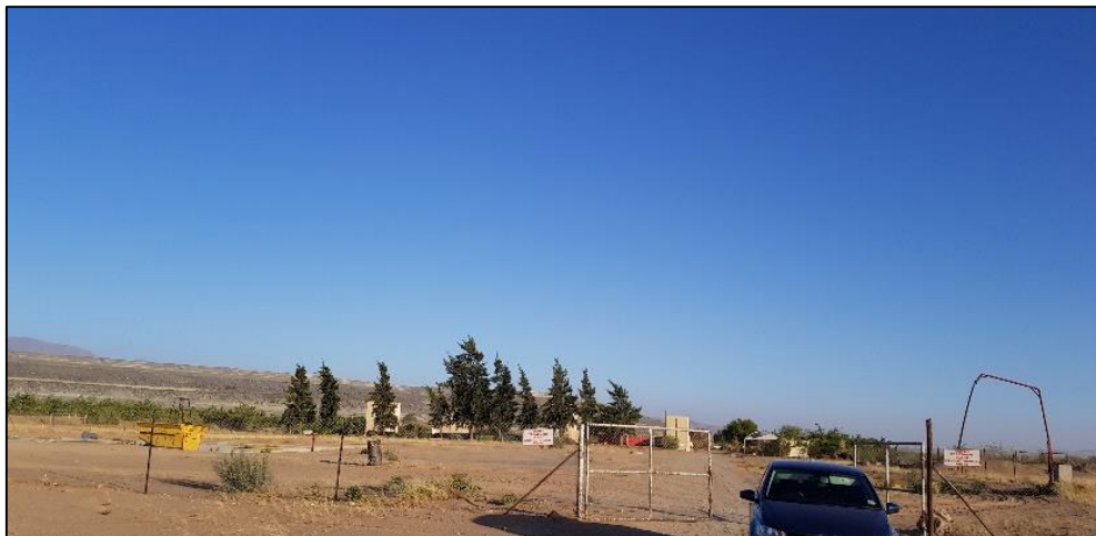
Figure 5: Entrance gate to the Sewage Treatment Plant
