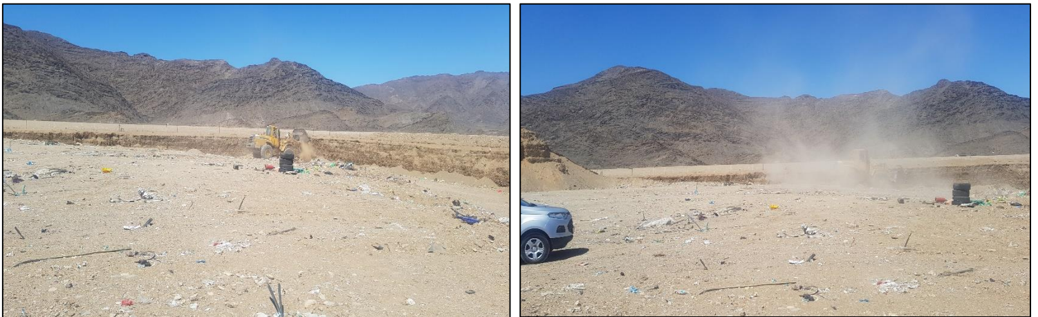
Figure 4: Waste being compacted in the process
