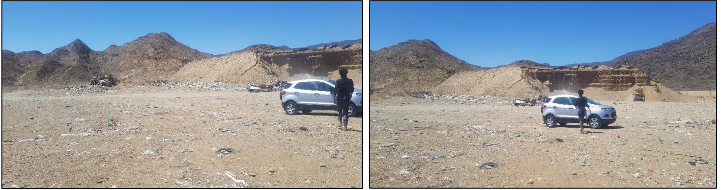
Figure 5: Heaps of sand excavated from cell 1 used to compact the waste
