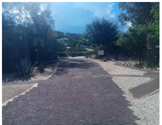
Photo 17: Paved Internal Routes and Walkways
