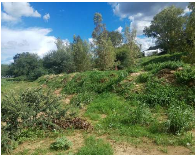
Photo 4: North to NE – Non-permanent Retaining Wall
